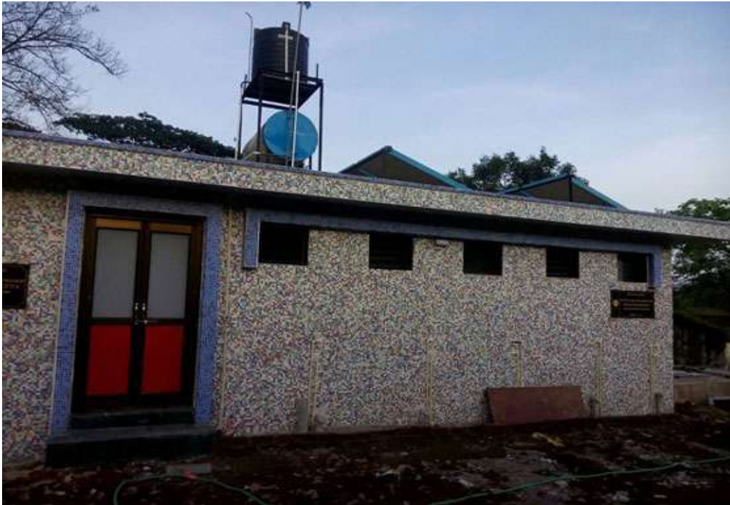
Toilets made for Villagers
